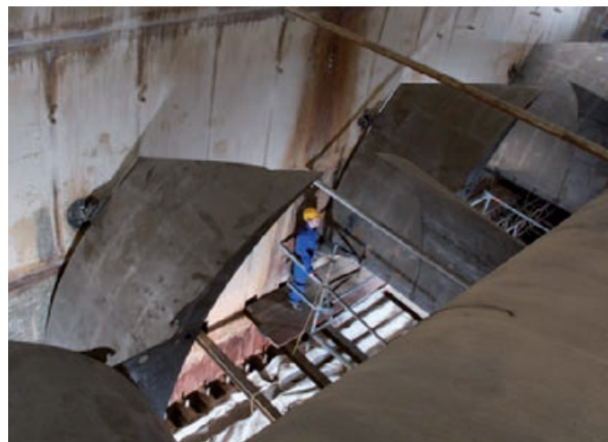
Installation of Sulzer Contour™ mixers in a large gas duct
